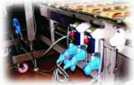
Deconnectors with optional pilot contacts can convey alarms or control auxiliary equipment along a conveyor line.
