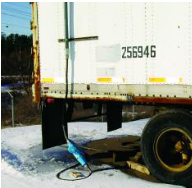
Decontactors provide convenient power supply connections and local disconnects for mobile facilities.
