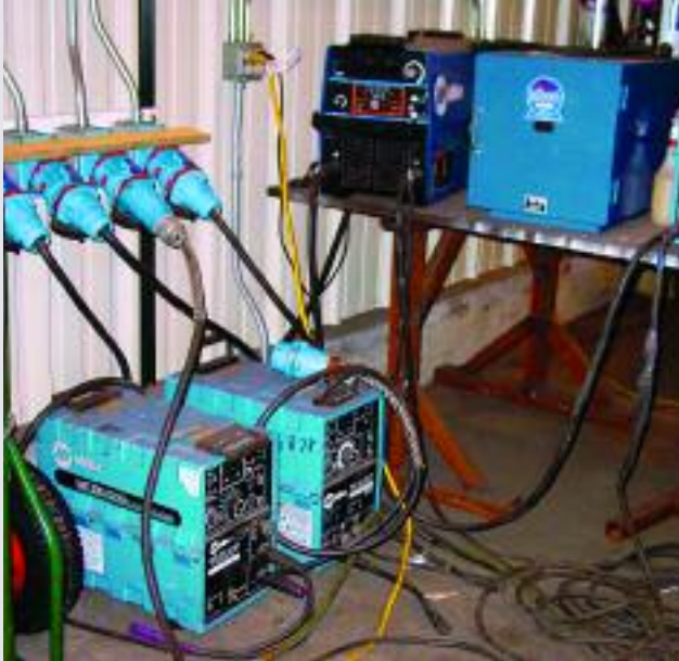
Decontactors allow welders to safely connect and disconnect welding machines even under overload conditions.
