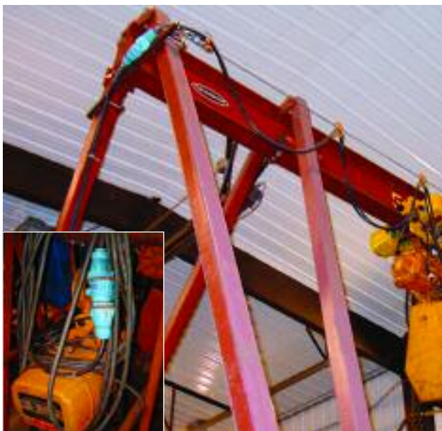
Deconnectors used as in-line disconnects facilitate quick and safe servicing of hoist equipment.
