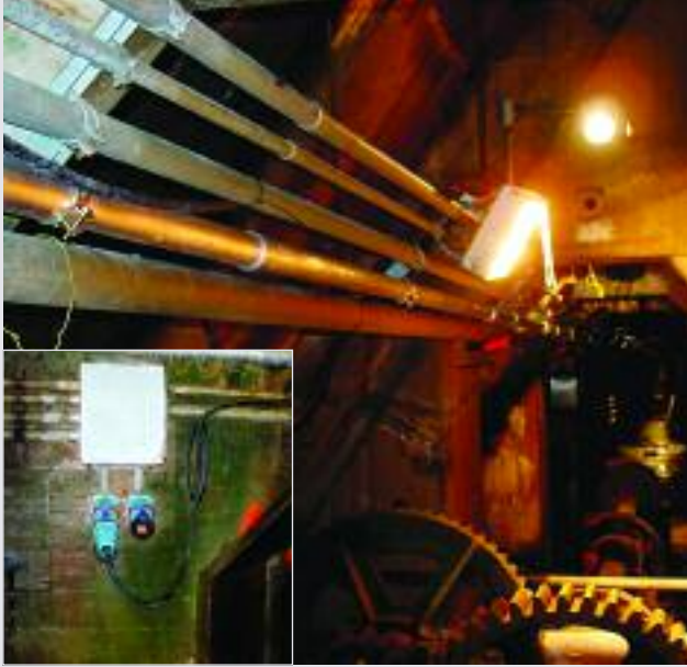
Meltric plugs and receptacles ensure worker safety when connecting heat lamps or other lighting loads, even in damp conditions.
