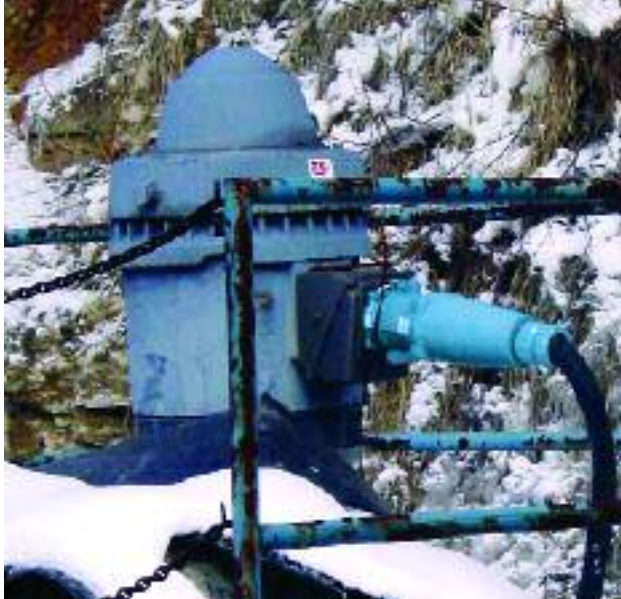
A 200A, NEMA 3R rated DS Series DECONTACTOR connects power to a float pump via a direct mounting configuration. When required, the DS receptacle is disconnected and the pump is easily relocated to another retention pond.
