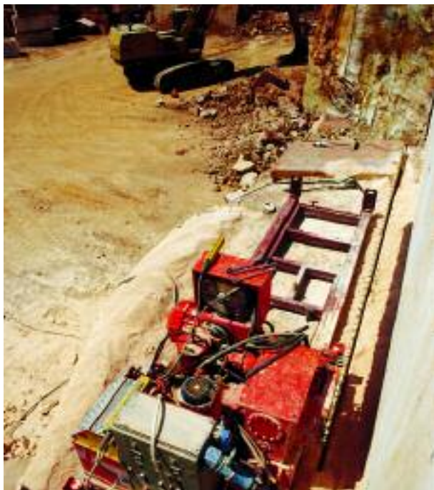
Meltric DS devices supply power to large cutting machines at a marble quarry. DS's are UL and CSA switch rated, allowing them to function as a 'line of sight' disconnect.
