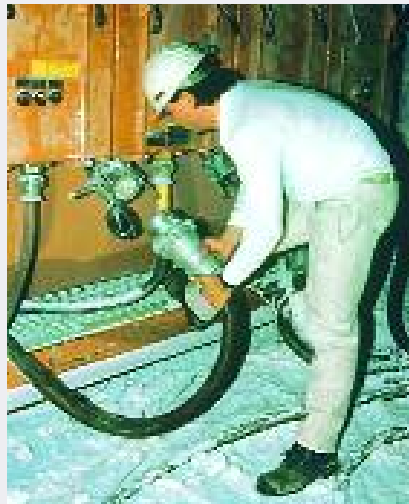
Mobile generator at salt mine
