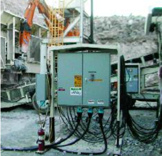
200A DS200's distribute power from portable generators to a power distribution panel (pictured) and then to conveyors and other electrical equipment. A DSN24 Multipin connector (left of the panel) provides control wire connections to the PLC cabinet in a single convenient connector.
